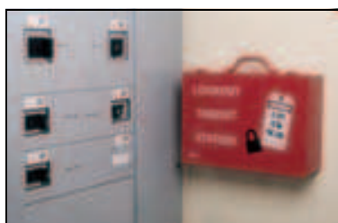
Mount close to power and distribution panels
